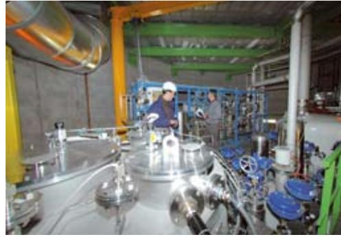
The CCS refrigerators are installed in cavities around the LHC.
