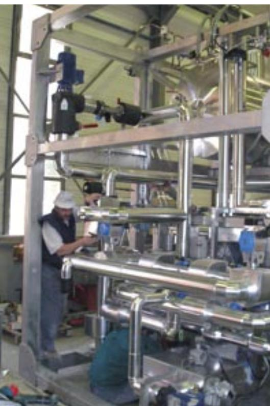
In the plant, a technician during the assembly phase of thermal isolation on the integrated ductwork.
