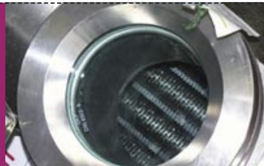
Accumulated solvents and water solidified on the tubes of a cryo-condenser
